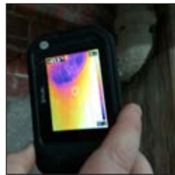
Thermal imaging to detect water leaks, moisture seepage, and structural integrity (Photo: Rhonda Rinehart)
