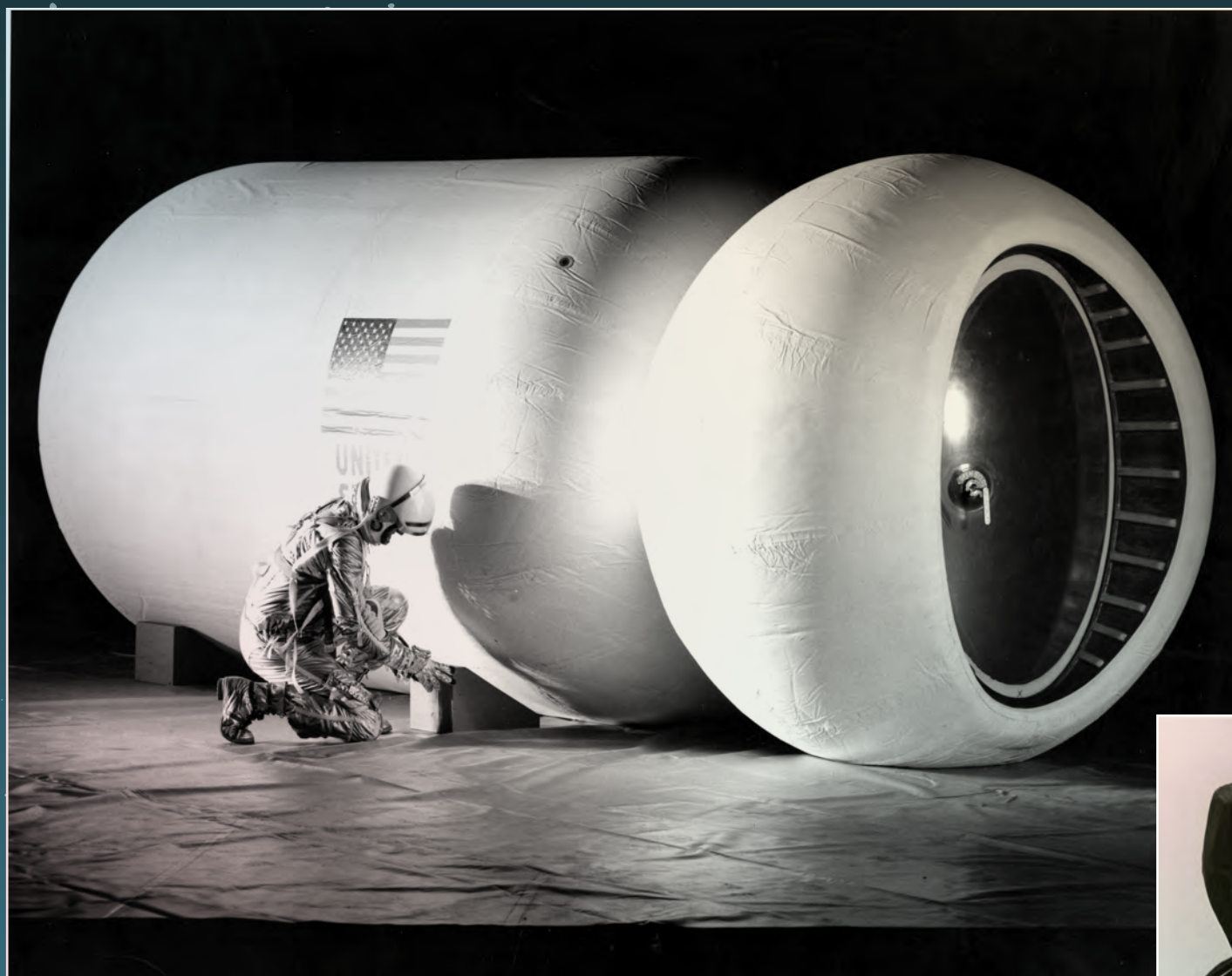
The Moon House, fabricated for NASA by the Goodyear Aerospace Corporation, was to provide future moon explorers with a home base for up to eight days. Goodyear Tire and Rubber records, 1969, University of Akron, University Libraries, Archival Services.
