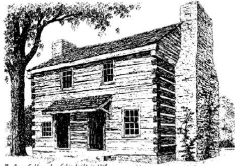
The James Galloway Log Cabin built in 1796, a part of the Greene County Historical Society Complex.
